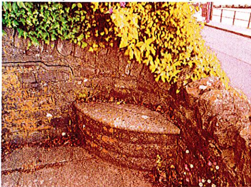
P7: The Spa. Steep vegetated bank (left) and displaced concrete footpath with uneven surface. The hand rail is slightly bent. Cracks on footpath have been covered with concrete painted with yellow colour. Looking south.
