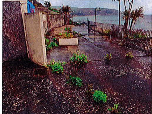
P24: Spa Beach Huts. Fairly good condition of steps and retaining walls. It can be assumed that the prefabricated concrete block wall (right) was built before the natural stone blocks wall (left). Looking west.
