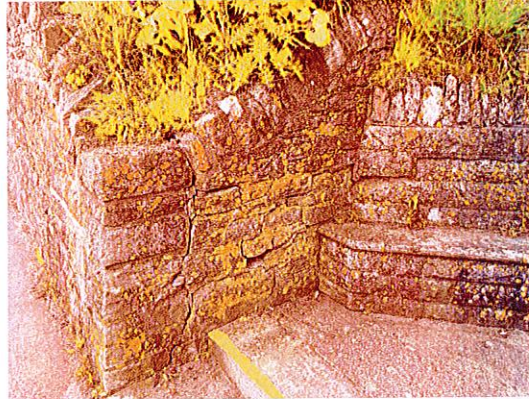
P4: The Spa. Retaining wall (0.5-1.0m high) showing a vertical crack and minor tilting eastwards. Looking sothwest.
