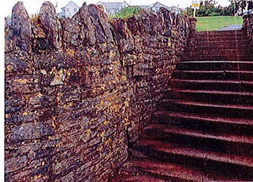
P48: Sandpit Field. Retaining wall (≈1-1.5m high) with localised vertical crack. Looking west.
