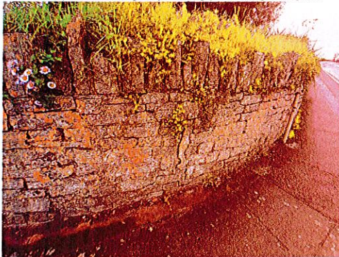
P47: Sandpit Field. Retaining wall (≈1-1.5m high) with cracking. Looking west.
