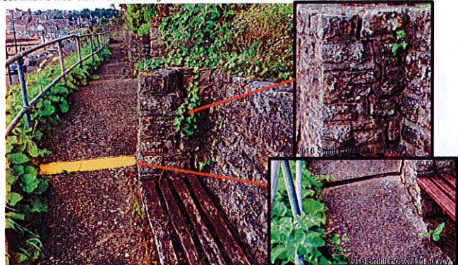
P8: The Spa. Steep vegetated bank (left) and displaced concrete footpath with uneven surface. The hand rail is slightly bent. Cracks on footpath have been covered with concrete painted with yellow colour. Retaining wall showing a vertical crack which is wider than in 2016. Looking south.
