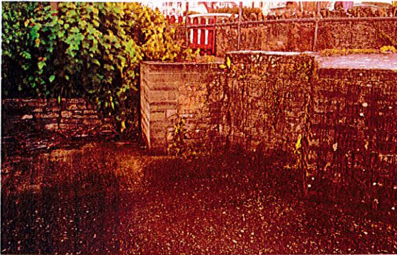
P23: Spa Beach Huts. General aspect of retaining walls with various retained heights (≈0.5-1.5 m high) along the western section. Partial reconstruction of existing masonry wall made of natural stone blocks using prefabricated concrete blocks noted at the centre of the image. Seepage on the walls is due to heavy down pour occurring at the time of the visit. Looking northwest from within the site.
