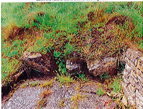
P43: Sandpit Field. Partially collapsed retaining structure ( \approx 0.5\text{m} high). Backfill pushing eastwards has knocked down the natural stone blocks. Looking west.
