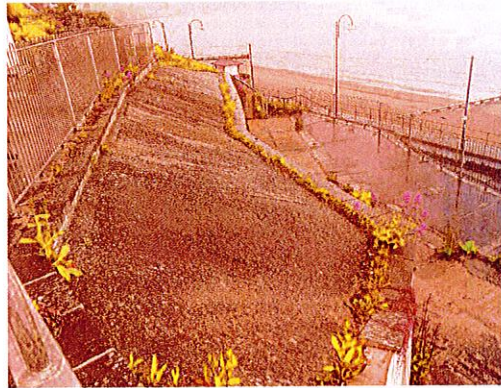
P20: Spa Beach Huts. Concrete slabs with repairs sloping eastwards and supported by a retaining wall ( \approx 2\text{--}2.5\text{m} high). Presence of steel railings across perimeter. Concrete repairs evident on the lower level (right). Looking northeast.
