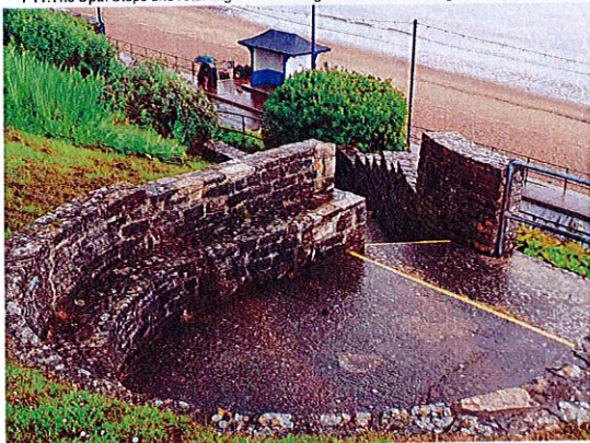
P11: The Spa. Steps and retaining walls showing some minor cracking. Looking northeast.
