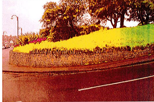
P50: Sandpit Field. General view of Sandpit Field eastern retaining wall with localised cracking. Looking south.
