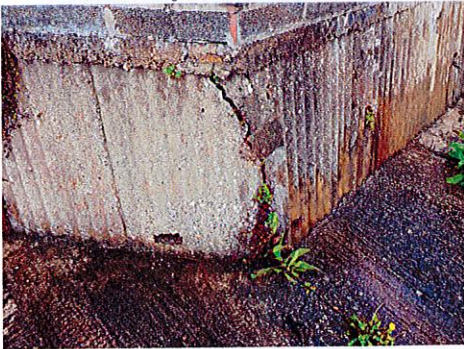
P27: Spa Beach Huts. Detail of vertical crack across the base of the retaining wall comprising prefabricated concrete blocks (above) over concrete with wavy patterns vertically oriented (below). Some of the weep holes are partially blocked with vegetation and sediments. Looking west.
