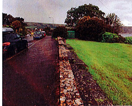
P16: The Spa. Grassed slope gently sloping eastwards. Retaining wall supporting De Moulham Road and defining the western site boundary. Pavement (left) is uneven. Looking north.
