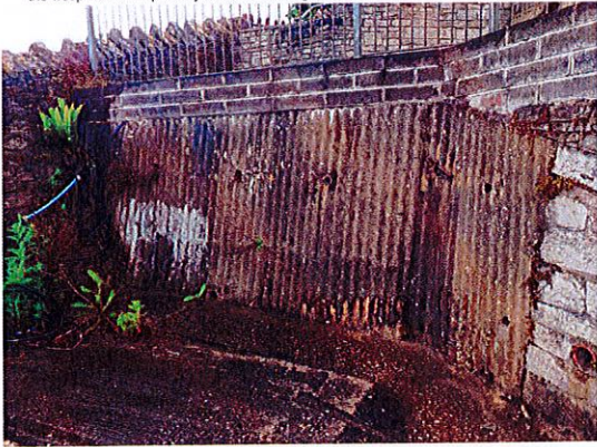
P27: Spa Beach Huts. Detail of vertical crack across the base of the retaining wall comprising prefabricated concrete blocks (above) over concrete with wavy patterns vertically oriented (below). Some of the weep holes are partially blocked with vegetation and sediments. Looking west.
