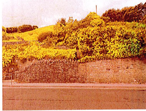
P4: The Spa. Retaining wall (0.5-1.0m high) showing a vertical crack and minor tilting eastwards. Looking sothwest.
