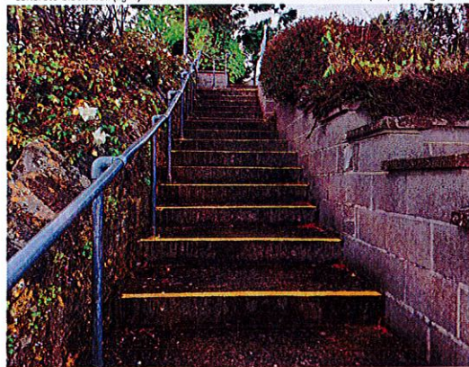
P24: Spa Beach Huts. Fairly good condition of steps and retaining walls. It can be assumed that the prefabricated concrete block wall (right) was built before the natural stone blocks wall (left). Looking west.
