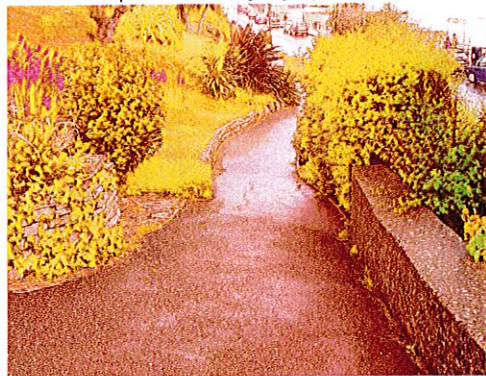
P44: Sandpit Field. Partially collapsed retaining structures ( \approx 0.5\text{m} high). Backfill pushing eastwards has knocked down the natural stone blocks. Looking northwest.
