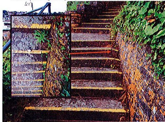
P8: The Spa. Steep vegetated bank (left) and displaced concrete footpath with uneven surface. The hand rail is slightly bent. Cracks on footpath have been covered with concrete painted with yellow colour. Retaining wall showing a vertical crack which is wider than in 2016. Looking south.
