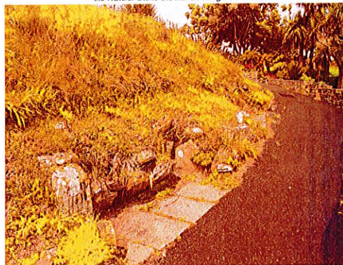
P44: Sandpit Field. Partially collapsed retaining structures ( \approx 0.5\text{m} high). Backfill pushing eastwards has knocked down the natural stone blocks. Looking northwest.
