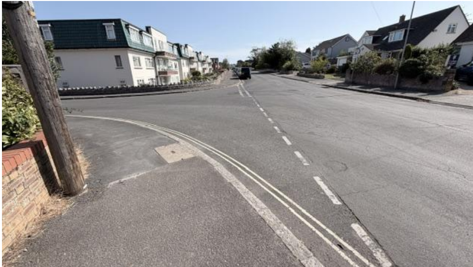
No drop curbs on this junction
