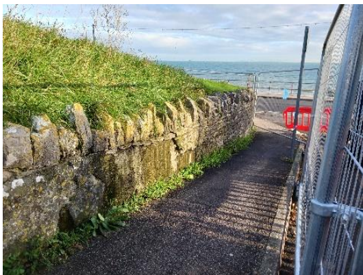
Image 4 and 5: Signs of ground movement on walls around the Green Seafront – Credit – Dorset Coast Forum
