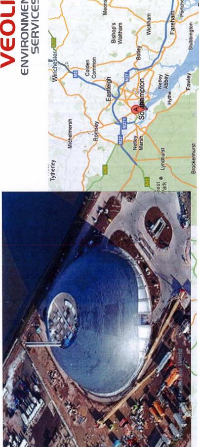
metals are extracted for recycling and the plant provides electricity for 20,000+ local homes. This plant achieves ~80% diversion form At least 4,000 tonnes of rubbish per year is sent to the Energy from waste plant in Southampton operated by Veolia. Some andfill. This contract is due to expire in August 202′
