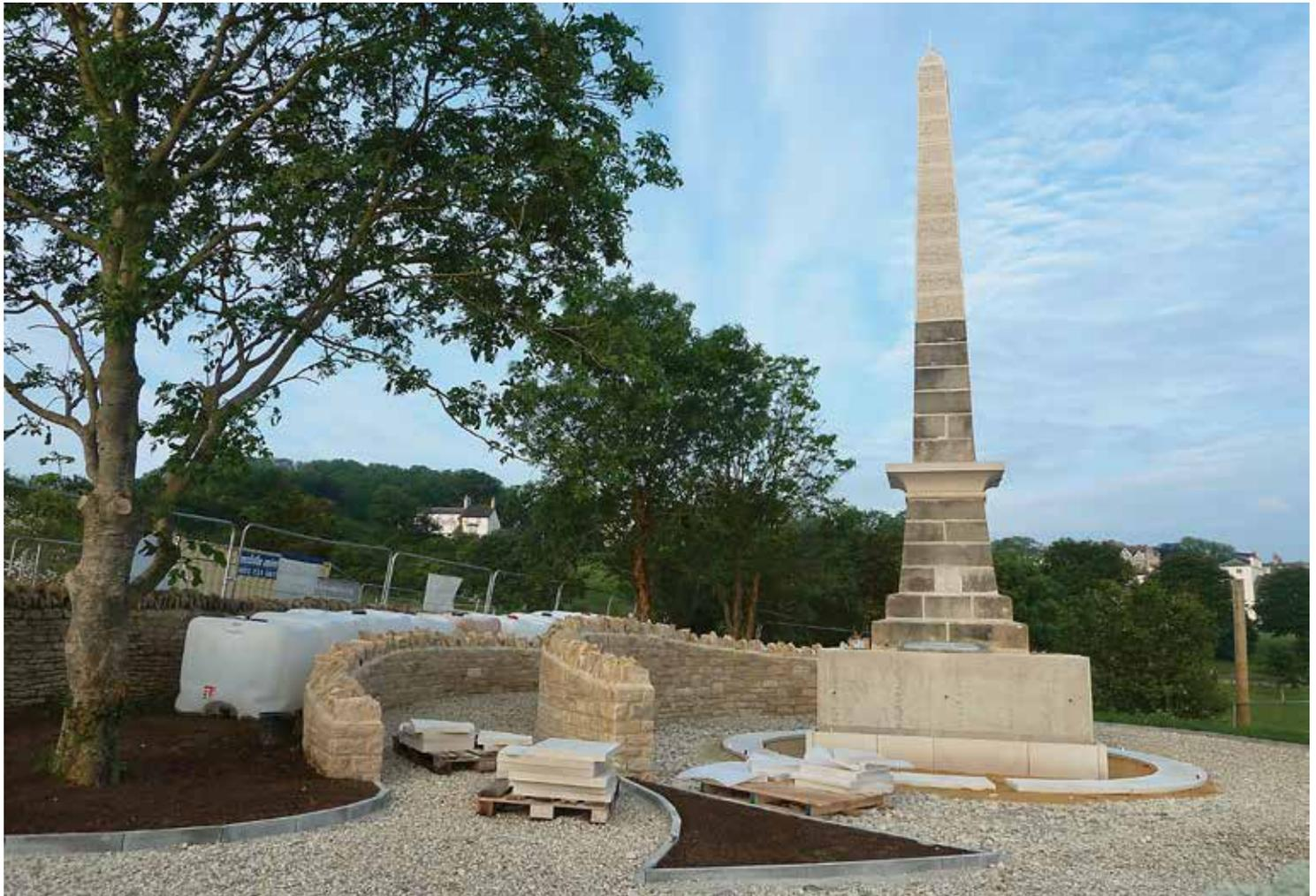
The reconstruction of the original Prince Albert Memorial is now reaching its finale with only the finishing touches - the stone facing of the plinth, the railings with corner supports, paving and surfacing of the paths, benches and planting - needing to be completed.
