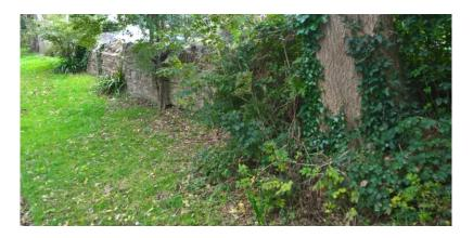
The earth banking against the inside of the wall will be removed but retained on the Downs. The earth will be placed in a nearby "dip" in the landform to minimise the impact. This will avoid landfill costs and is the most sustainable option as there is minimal transport and any viable seed bank held within the topsoil is retained on the Downs.
