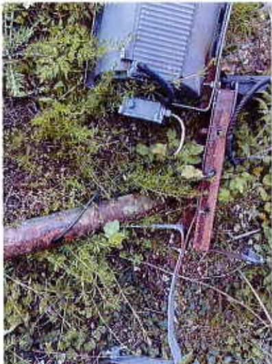
Rotten electrical cabinets and poles.
