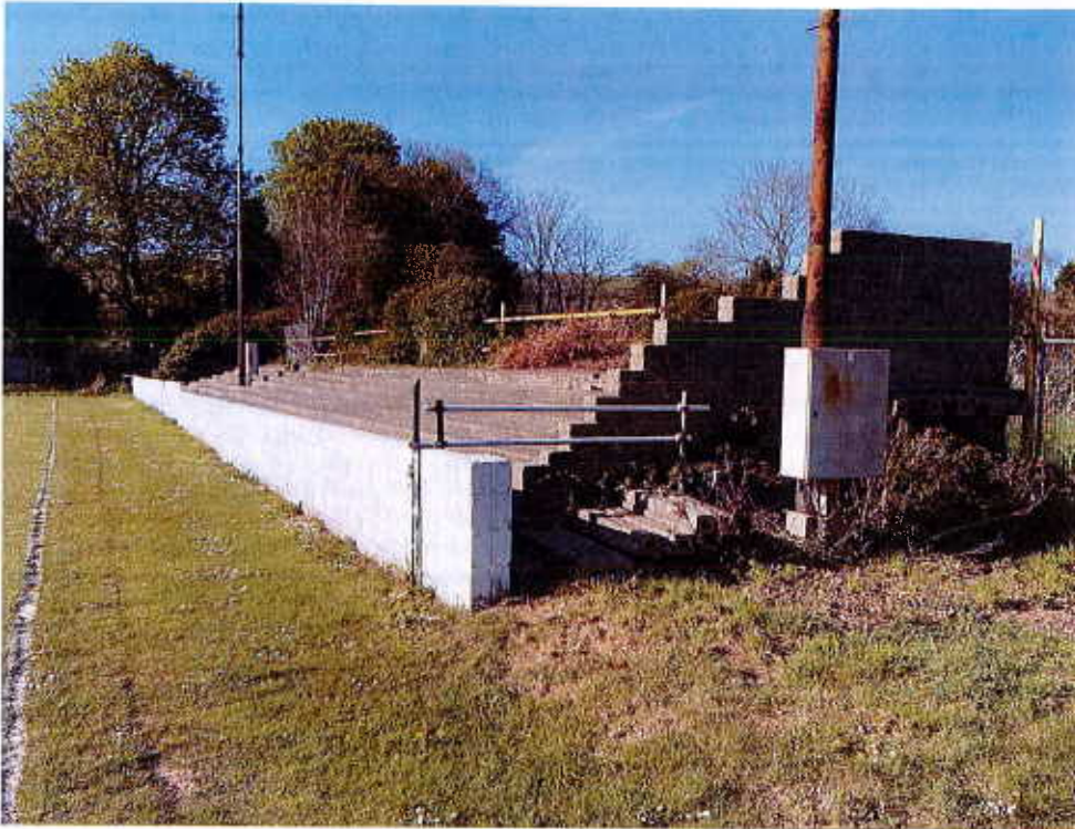
Concrete stand to be demolished to make way for 5 aside pitch.
