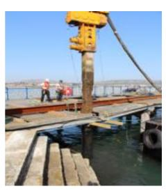
This photo shows an old pile being extracted - note the middle section showing how it has rotted away. The photo at the top is of a new pile being driven in.
