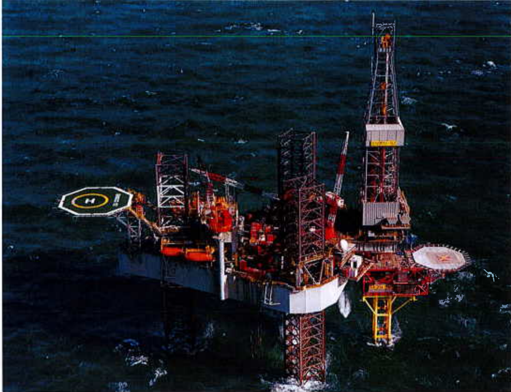
Figure 3.2. Indicative Jack-up Drilling Rig (Ensco 92) (ENSCO Plc, 2017)
